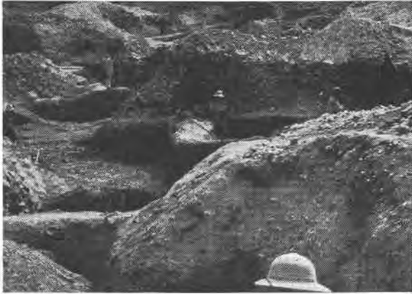
FIG. 6. Pits in shale, some of which extend down to lower bull quartz horizon, Mimoso, Baia. Walls of broken rock between pits are shored up with boulders of bull quartz which have been mined in search for crystal. Stripping has exposed upper quartz horizon in left center of the photograph. Man in center stands on top of upper quartz horizon.
