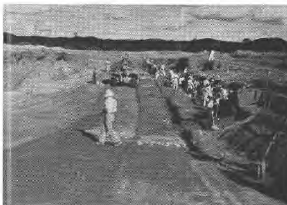
FIG. 11. Prospect pits in residual weathered rock representative of the hundreds of such pits near Sete Lagôas, Minas Gerais. The bedrock in this region is red shale. Rock fragments are bull quartz.
