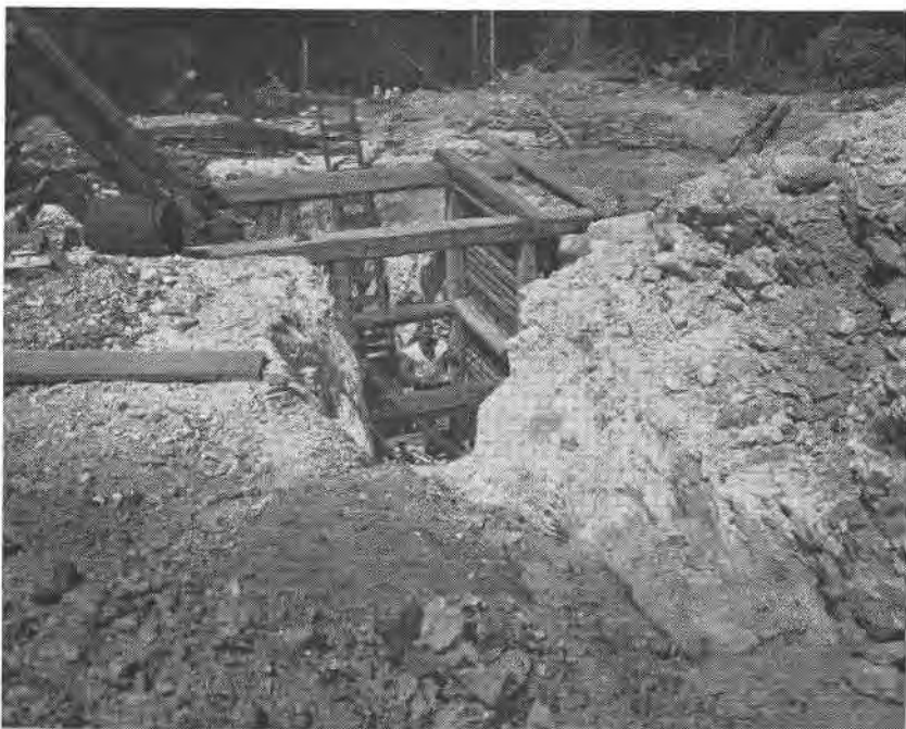
FIG. 5. View of shaft and part of main open cut, Pidlite mine, looking northeast. The openings are in lepidolite-rich pegmatite. Massive quartz with blocky fracture is exposed high on wall of cut at right.
