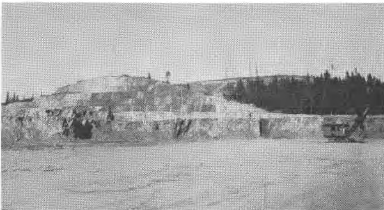
FIG. 1. The upper benches of the Zonolite mine at Libby, Montana.
