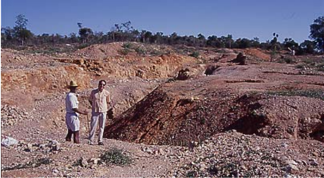
Photo 1 – View of the works at Anjahamiary in November '00, showing the trench along the core-zone of the pegmatite. Photo Federico Pezzotta.
