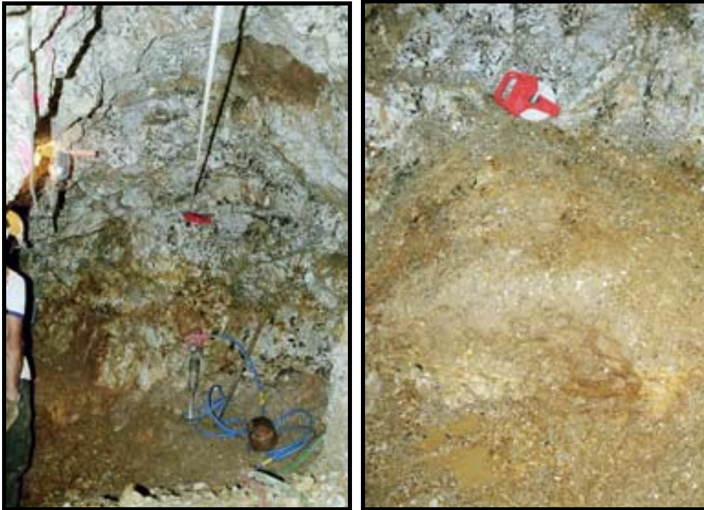
Figure 36: Continuation of the Working face, N 20 W. The face of the wall for File 104 has been removed for a distance of about 30 cm. Figure 37: Top of Pocket, File 104, exposed on 8/8/03. This zone is shown as the anomalous regions in File 104 in Figure 23, as the sloping line just before marker 1m and ending just after marker 2m, and as the angled line of bright energy zones between markers 1m and 2m in Figure 24. Additional bright energy zones are now clearly shown between markers 1m and 2m at 1.35m depth, and at marker 3m at 1.15m depth.
