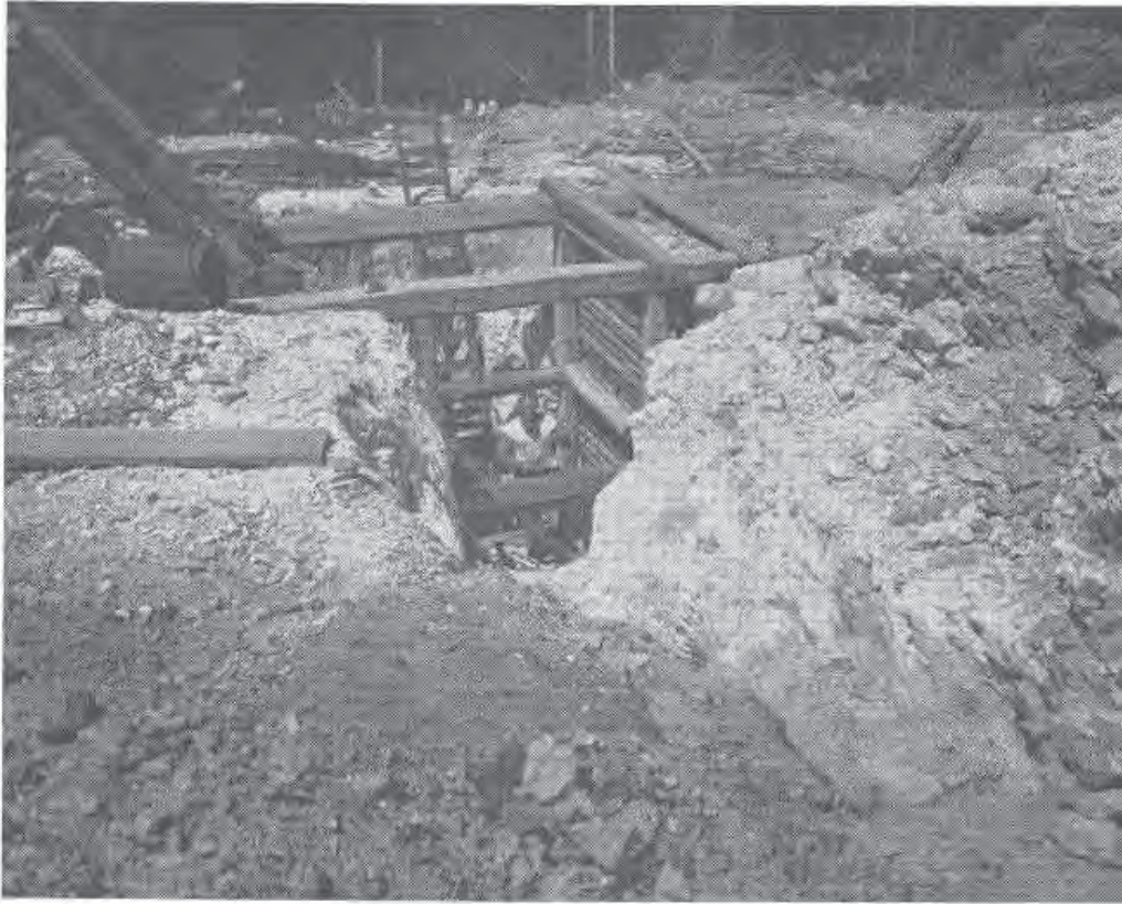
FIG. 5. View of shaft and part of main open cut, Pidlite mine, looking northeast. The openings are in lepidolite-rich pegmatite. Massive quartz with blocky fracture is exposed high on wall of cut at right.
